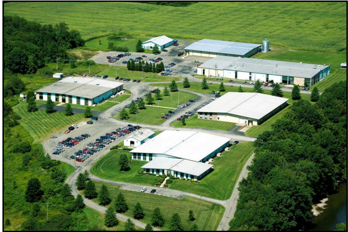
Facilities in Saegertown, PA
